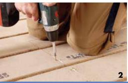
Joist structures: when using Novopan's grooved return panels, a stub joint will occur in each row of panels (where the tongue-and-groove has been sawn off – a rubbed joint). These panels must always be joined over a joist.
